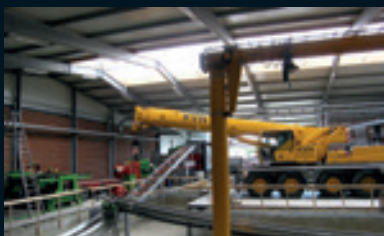
Installationsarbeiten zu neuen Pressenlinien Installation works carried out for new pressing lines
