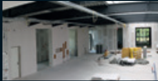
Innenausbau des Besucher-Zentrums Interior finishing of the visitor centre
